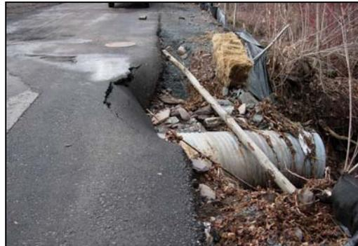
Stormwater runoff from Garfield Road east of the intersection with Point Breeze Drive and runoff from Prince and Lookout Mountain Drive currently discharge directly to the Schoharie Creek via a culvert underneath Route 23A. Within this drainage area there are five swales and five culverts that represent potential stormwater runoff sediment sources.
