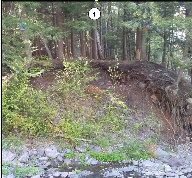
Looking at the west side of the railroad bed.
