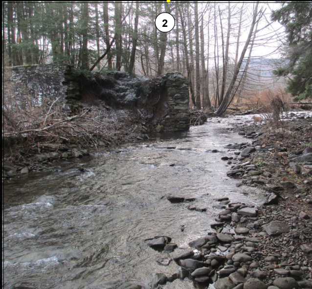
Looking south at the east abutment of the railroad bed.
